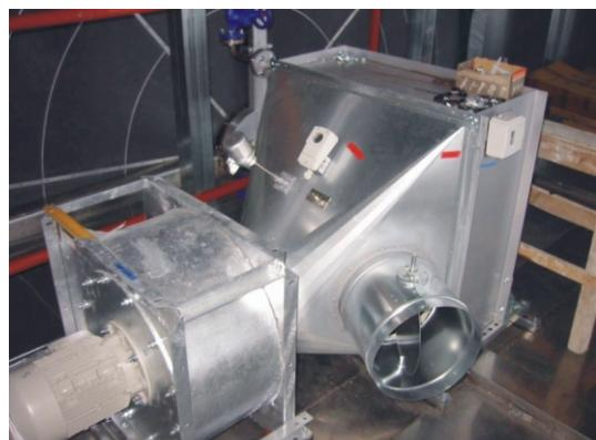
... and, through the connecting duct in the outgoing air section, blows it in the pulse chamber of the heat wheel in opposite direction of the exhaust air flow.
